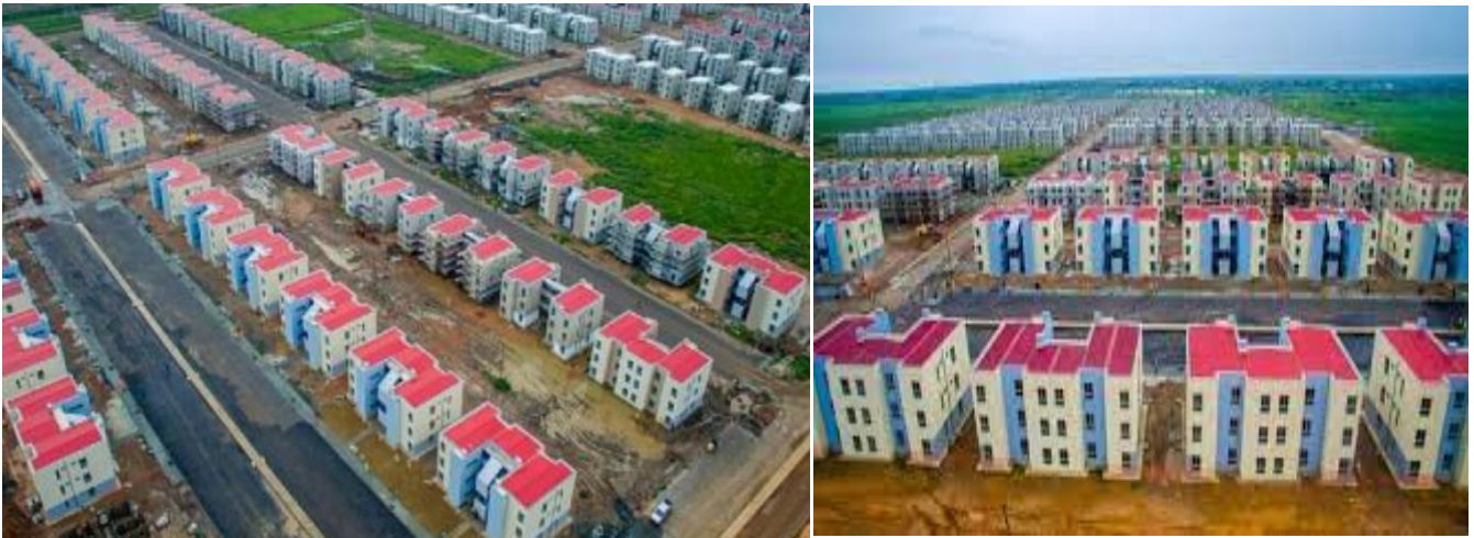
Figure 4.1 Pictorial view of the Saglemi Housing project
