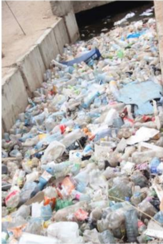
Figure 5.9: Plastic bottles blocking drain (Zehra et al, 2019)
